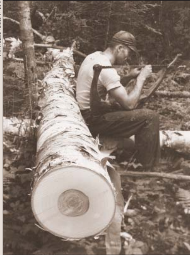
New Hampshire logger with saw, circa 1925. Trees were cut, sawed into 4-foot lengths and piled for seasoning. Previous page: Small stream driving harnessed waterpower to transport pulpwood to the paper mill. The Brown Company, Berlin, N.H.
