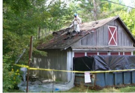
*Contractors removing asbestos roof shingles during the garage demolition at Union Meadows WMA in Wakefield.*
